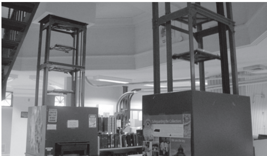
An automated conveyer belt system deep within the stacks of the Library of Congress.
